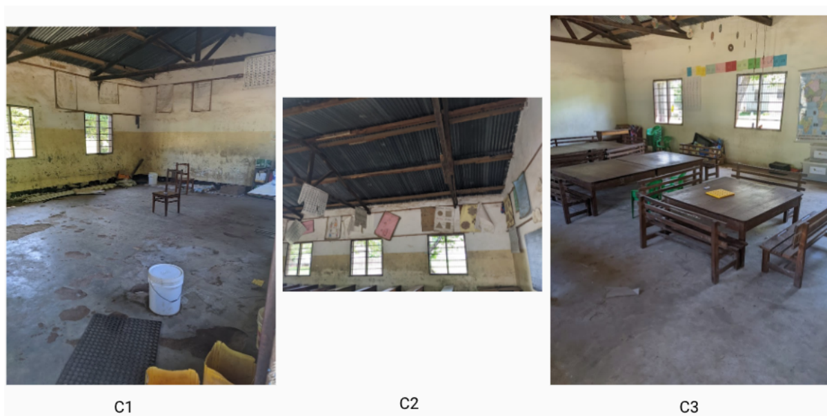
Figure 23: Author's picture of the three classrooms in the block which was investigated.
