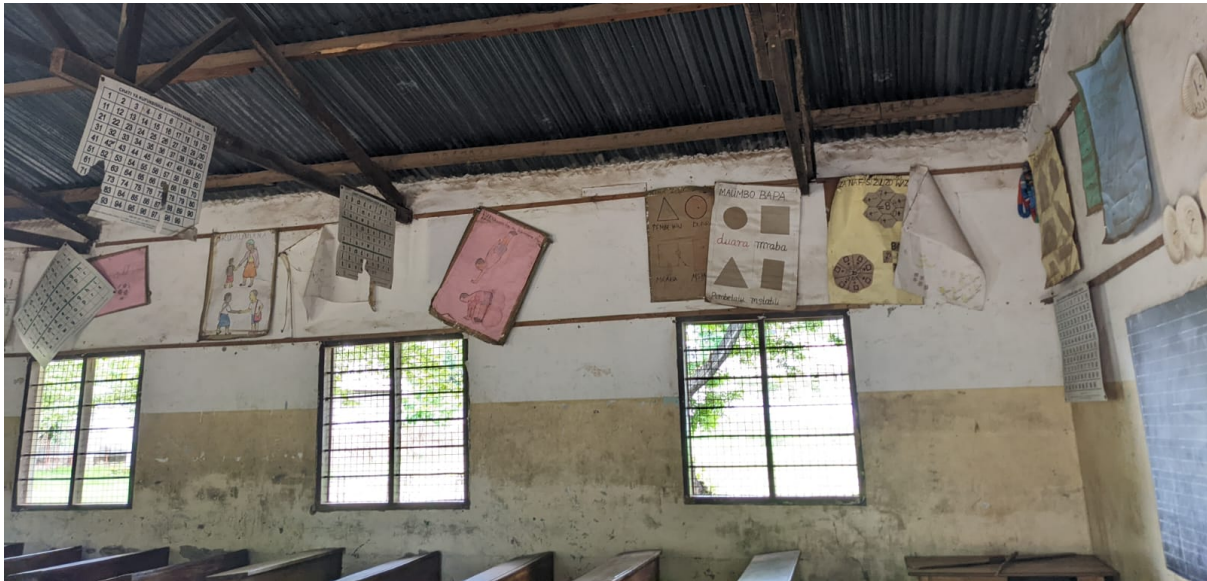
Figure 11: Shows the unglazed windows, which are common across classroom blocks in Tanzania.
