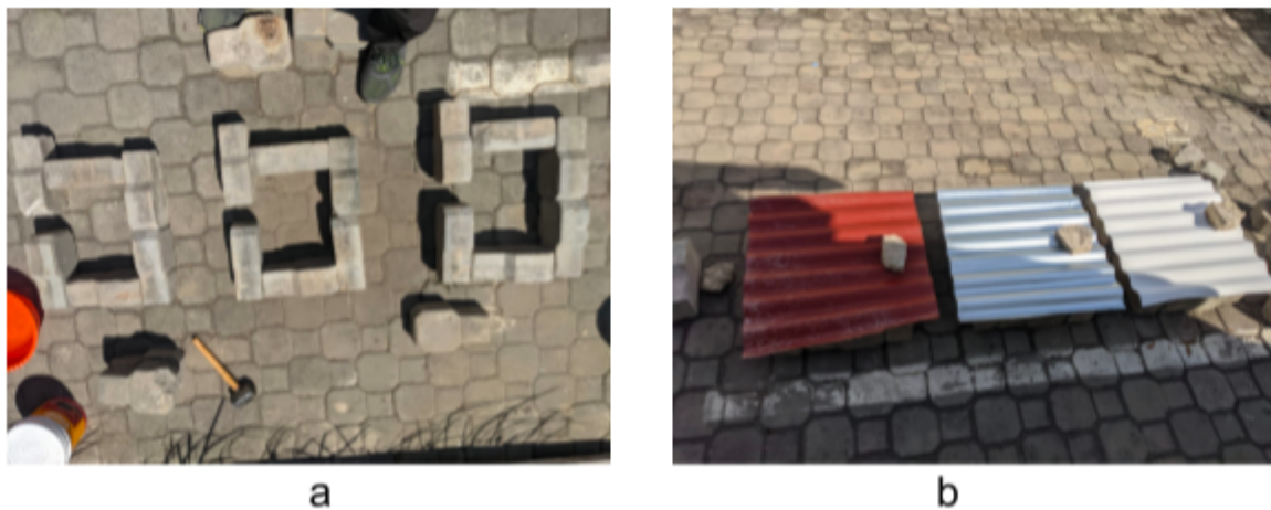
Figure 18: Showing the model classrooms which were built. (a) shows the bricks and (b) shows the models with roofing sheets.
